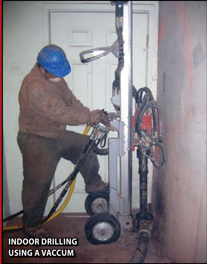
PRE-DRILLING FOR RESISTANCE PIERS
